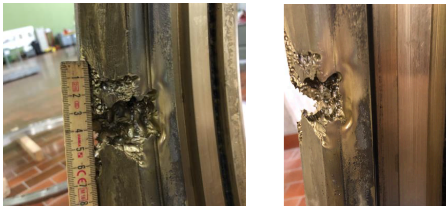
Picture of damage to a sealing ring of a ball valve due to a permanent water stream resulting from a leak eroding the sealing ring.
